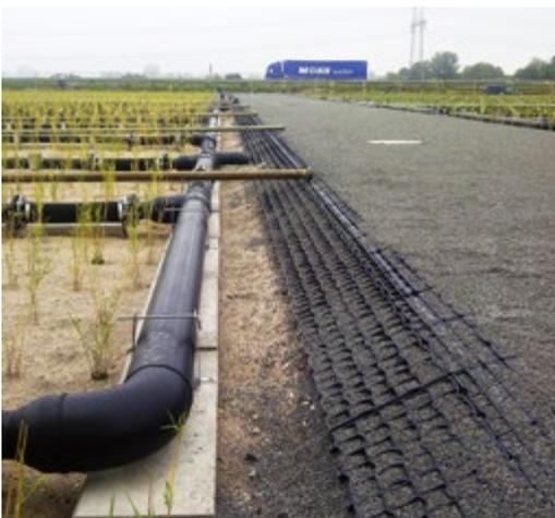
*"We used the ECORASTER® system for navigable reinforcement of the central embankment between the different plant beds and the circumferential dam - it has proven to be the best possible solution for our requirements: simple and quick installation by our own staff, smooth adaptation to the existing terrain, navigability by heavy agricultural vehicles and a truly cost-effective alternative."*
