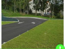
Keep the soil level just below the top of the ECORASTER® to protect the germinating seeds and ensure a durable parking/driving surface.
