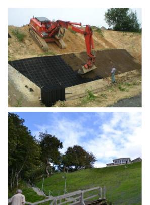
With over 200 expansion joints per square meter and 36 notched interlocking connectors per square meter the ECORASTER<sup>®</sup> counters the forces which are impacting the embankment. Erosion of the solum, soil destruction e.g. by rainwater made channels, line-shaped erosion and nutrient washout can be prevented by a proper installation of the ECORASTER<sup>®</sup> system.
